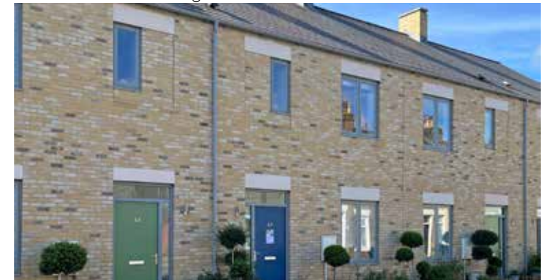
Flat fronted terrace with stone detailing
