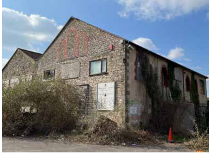
View east of existing Gasworks building
