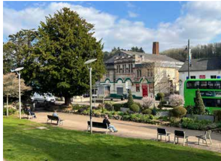
The building viewed across the Hollies Gardens
